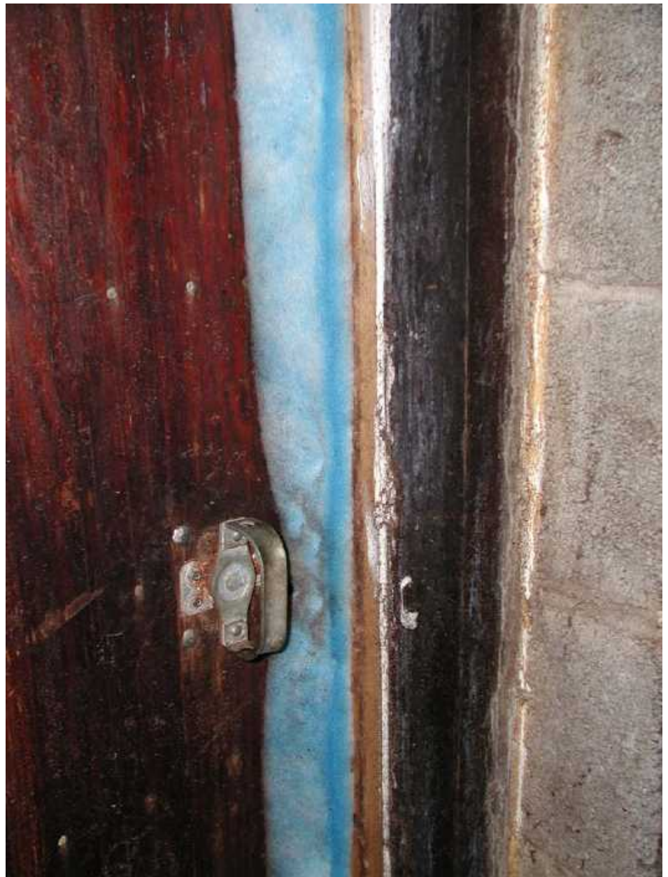
Figure 11. Filter material used to seal doors.
