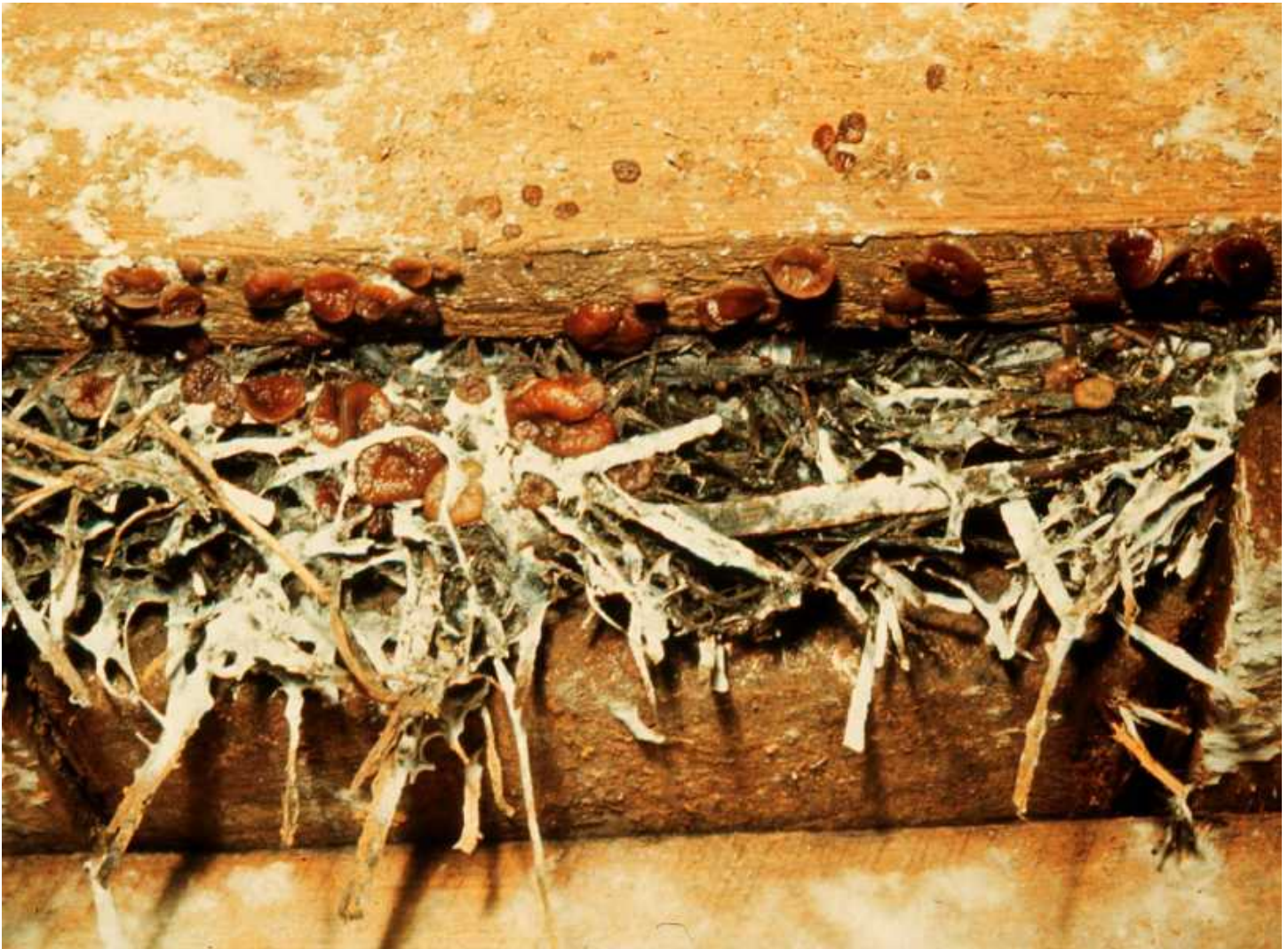
Figure 27. The cup-shaped structures caused by cinnamon brown mold have a rubbery or leathery texture and usually are dark brown, although chartreuse and yellow fruiting bodies have been observed.
