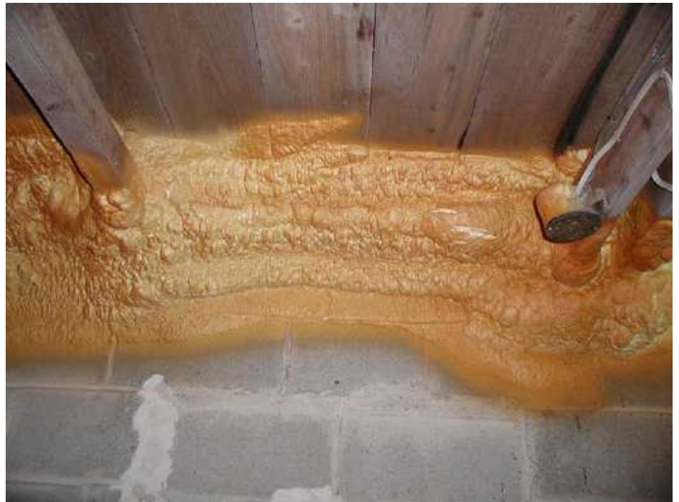
Figure 10. Rooms can be sealed with urethane insulation.
